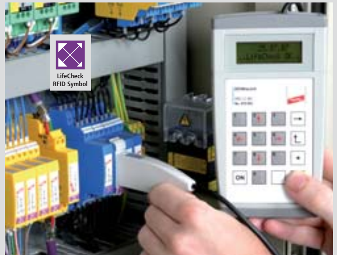
Testing an SPD module for use in intrinsically safe circuits (blue-coloured) by means of RFID technology (LifeCheck)
